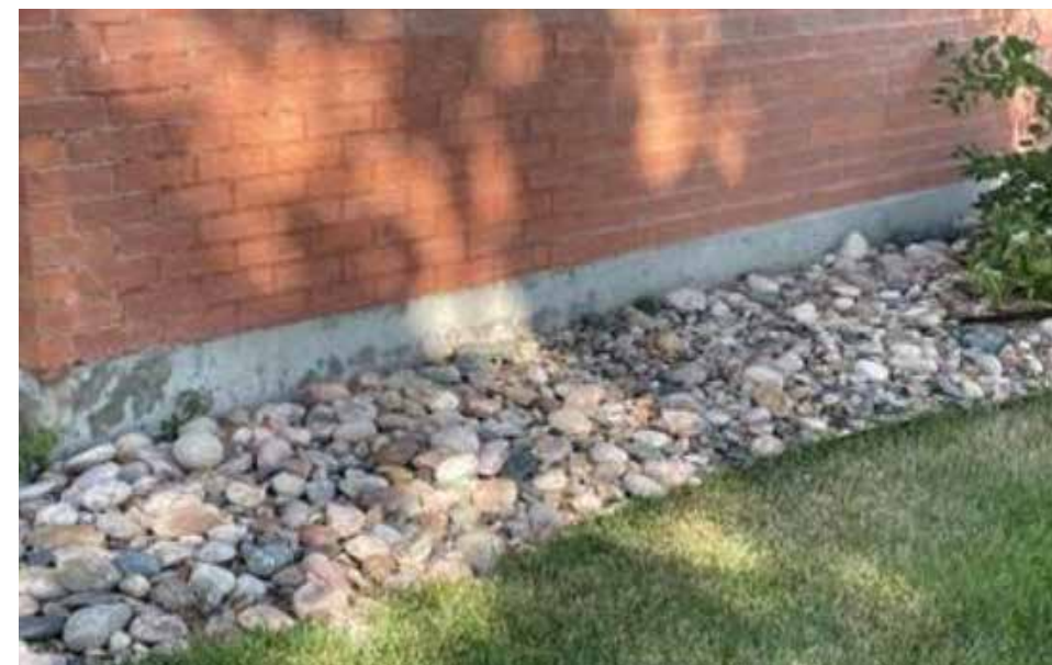
Figure 1.50b. Example of brick cladding. Brick cladding is one example of noncombustible siding that can be used. Image courtesy of Jensen Hughes/FEMA.
