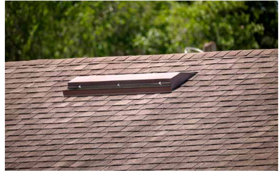
Figure 1.12. Off-Ridge vent. Off-ridge vents are typically best protected by having noncombustible screening.
