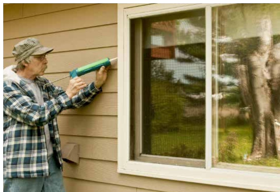
Figure 1.58a. Applying fire caulking around window-to-wall joints.
