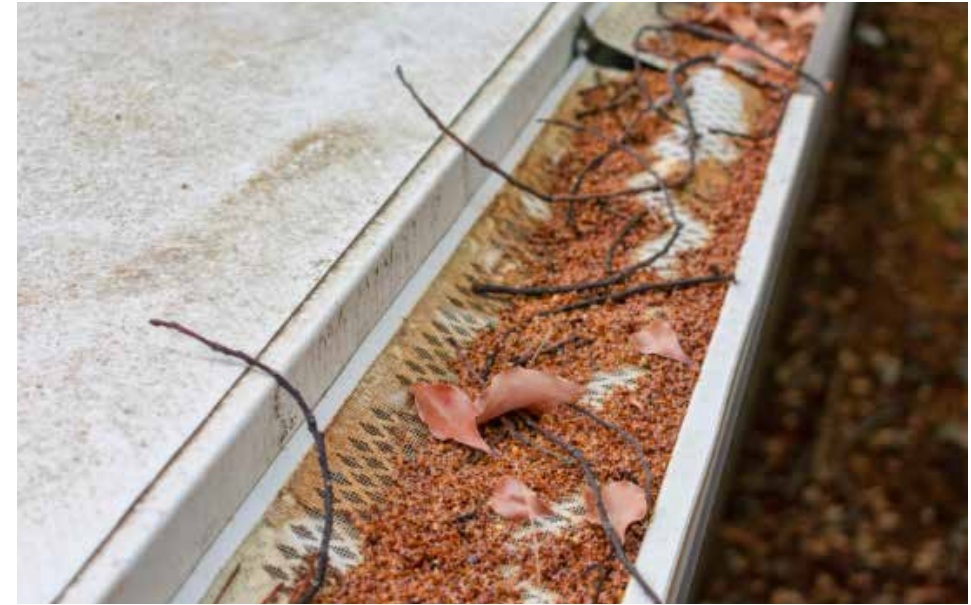
Figure 1.35. Debris accumulation on top of gutter guard. Notice that the guard is preventing debris from entering the gutter, but still leads to accumulation. This is evidence that roof edge protection is still necessary.
