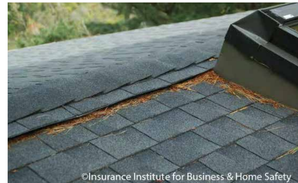
Figure 1.8. Example of roof ridge vent and collected debris. This accumulation of debris is vulnerable to ignition if not regularly cleared. If ignited, this burning debris would provide a flaming exposure to the plastic vent. Image courtesy of the Insurance Institute for Business & Home Safety.
