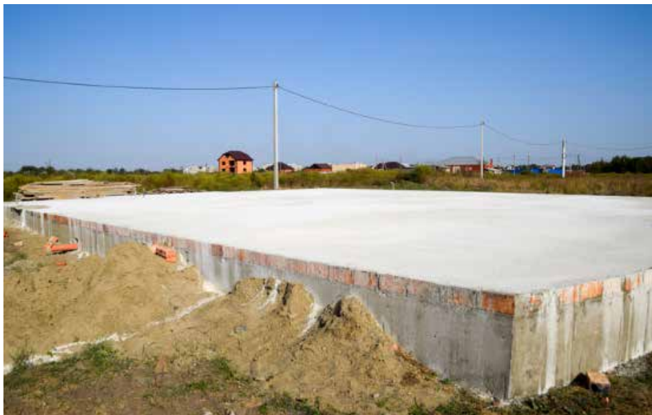
Figure 1.71. Mat foundation. Mat foundations are less susceptible to ember intrusion, however can be damaged in a fire event.
