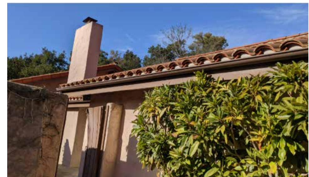
Figure 1.32. Sample bird-stopping at open ends of tiles at roof edges. Bird-stopping helps prevent debris accumulation and ignition of the roof. Image courtesy of Jensen Hughes/FEMA.
