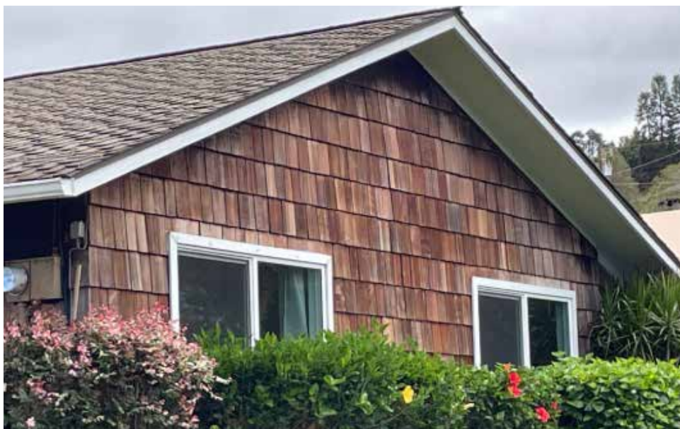
Figure 1.49. Example of combustible, wood shingle cladding on exterior wall, which presents a potential ignition hazard in a wildfire. Image courtesy of Jensen Hughes/FEMA.
