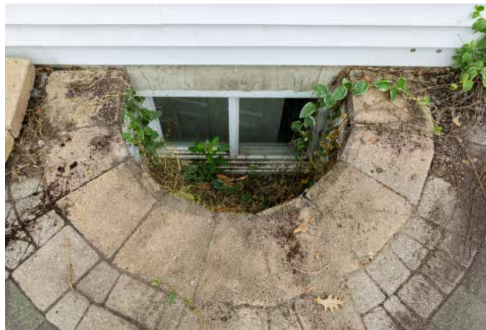
Figure 1.69. Example of unmitigated window well (debris collected at bottom, plants growing into and out of window well).
