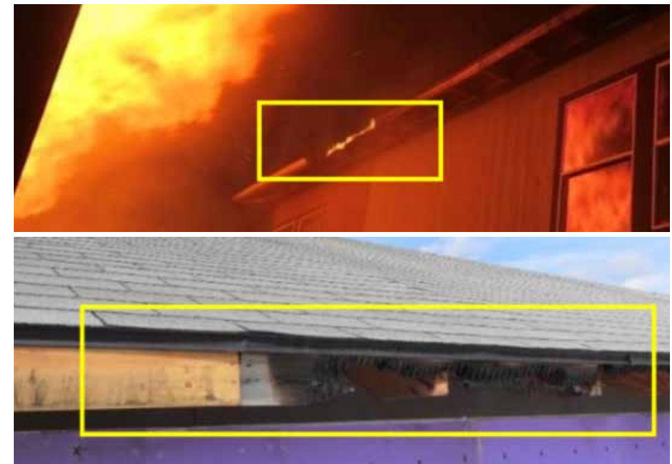
Figure 1.28a. (top) Vulnerabilities at roof edges (bottom) Fascia board ignition leading to roof joist ignition. These images demonstrate that gaps in the roof edge can lead to ignition of the structure. The top photo points to the contribution of the fascia in creating a “box” that can trap heat. Image courtesy of Insurance Institute for Business & Home Safety.
