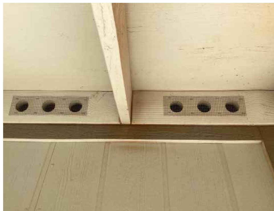
Figure 1.44a. Example of frieze block soffit vents with 1/4" metal mesh cover. Image courtesy of Jensen Hughes/FEMA.
