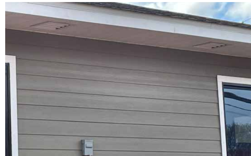
Figure 1.44b. Example of individual type soffit vents. Image courtesy of Jensen Hughes/FEMA.
