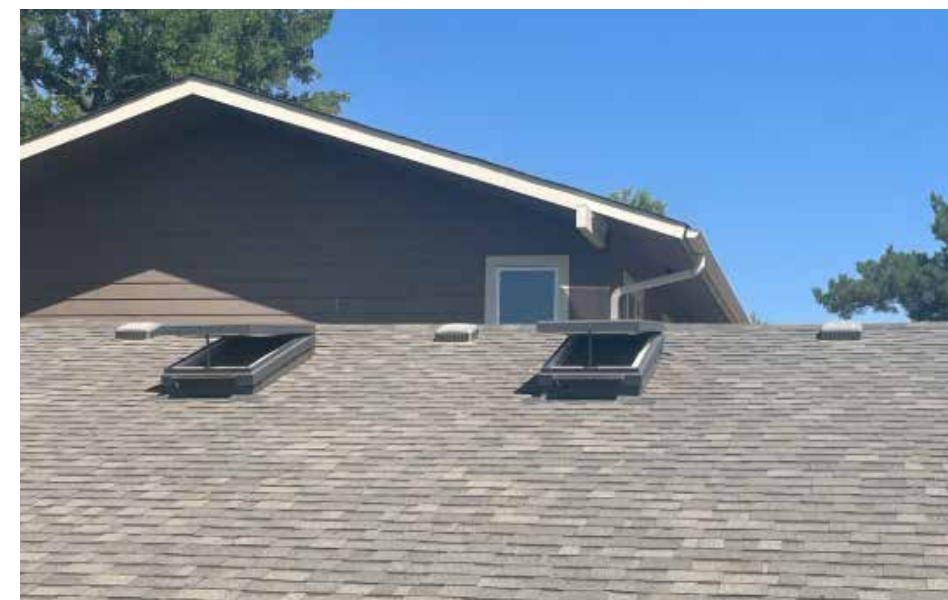
Figure 1.14. Example of the vulnerability of skylights when left open during fire events provide an unobstructed path for ember intrusion. Image courtesy of Commercial Roof USA.
