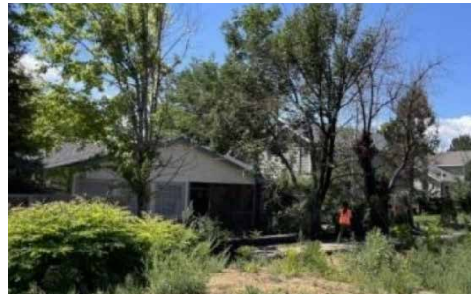
Figure 2.8a. Example of hazardous defensible space with overgrown vegetation overhanging and touching the structure, significant unmaintained trees, limbs, grasses, and shrubs in Zone 0 (0-5ft) and Zone 1 (50-30ft). Image courtesy of Jensen Hughes/FEMA.
