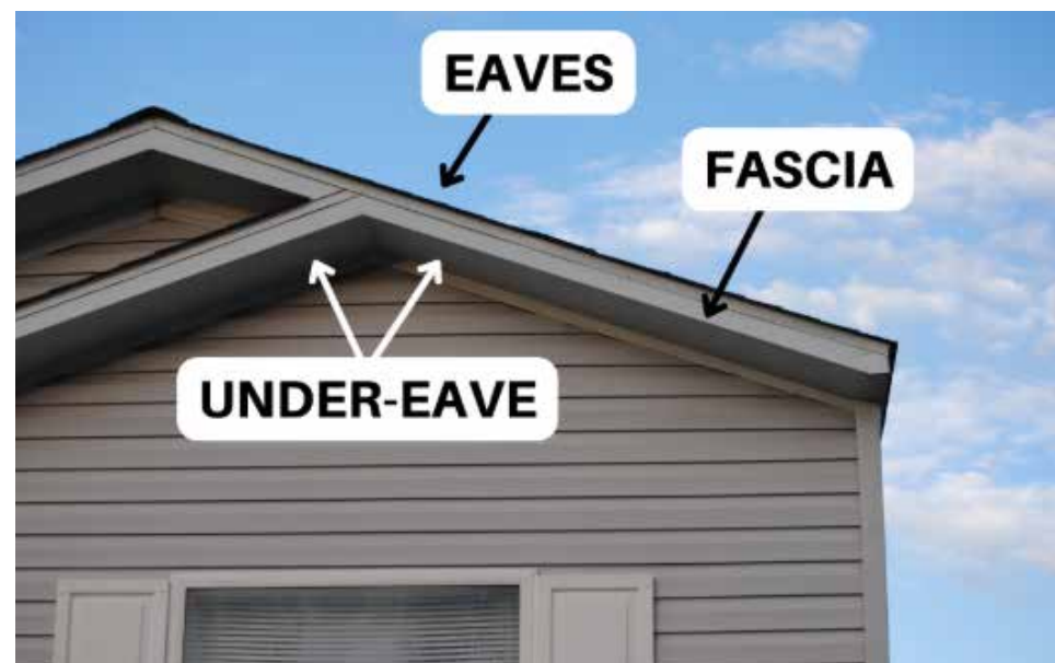
Figure 1.37. Structure showing the location of the roof eaves fascia, and under-eave areas. Under-eave areas can be soffited or open. Image courtesy of Jensen Hughes/FEMA
