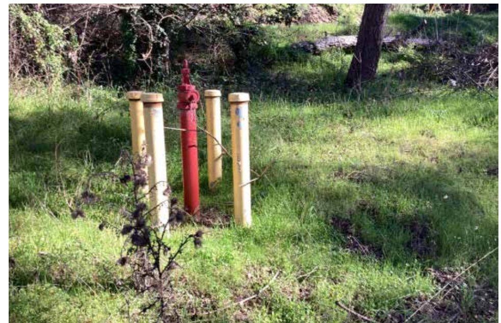
Figure 3.29. Fire department water supply connection. Image courtesy of Jensen Hughes/FEMA.
