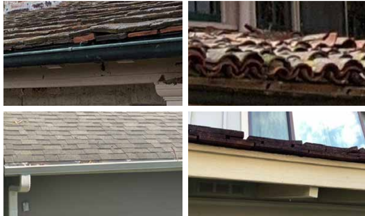
Figure 1.26. (top left) Weathered and poorly maintained cement tile roof with gaps and exposed wood shingles/sheathing; (bottom left) Asphalt shingles with metal drip edge, and proximate gutter with vegetative debris. (top right) Poorly maintained, barrel-shaped tile roof with large gaps and no birdstopping. (bottom right). Wood shingle roof edge with gaps and lack of metal drip edge detailing. Image courtesy of Jensen Hughes/FEMA.
