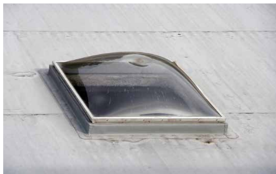
Figure 1.13b. Up close view of flat roof skylight with potential gapping between the skylight and the roof.
