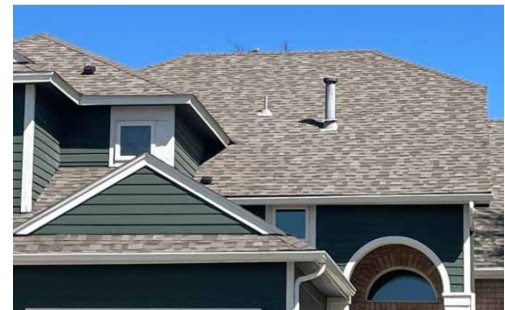
Figure 1.9. Example of through-roof vent. If not screened, through-roof vents can provide an avenue for embers to enter the home. Image courtesy of Jensen Hughes/FEMA.
