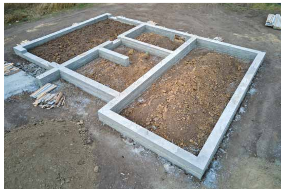
Figure 1.74. Example of wall footing. Footings can shift over time and create gaps along the interface of the foundation to the superstructure.
