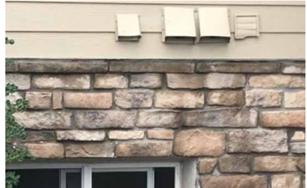
Figure 1.67. Example of dryer vent and other mechanical vents. When left unprotected, these can provide an entry point for embers into the home. Image courtesy of Jensen Hughes/FEMA.
