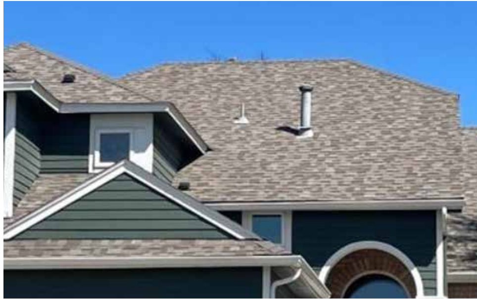
Figure 1.46. Example of a complex roof with several wall-to-roof joint conditions, which introduces locations for the collection of vegetative debris and embers. Image courtesy of Jensen Hughes/FEMA.
