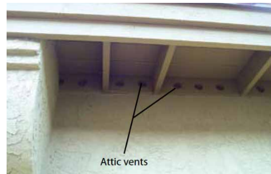
Figure 1.39. Example of open-eave construction, where the roof rafter rails are exposed and of combustible construction. Gaps between the blocking and rafter rails provide a pathway for ember entry. Image adapted from the. Image adapted from Home Builder's Guide to Construction in Wildfire Zones, FEMA, 2008. https://www.fema.gov/
