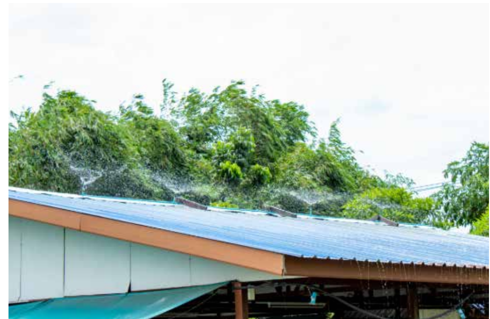
Figure 1.85. Roof provided with sprinkler system.
