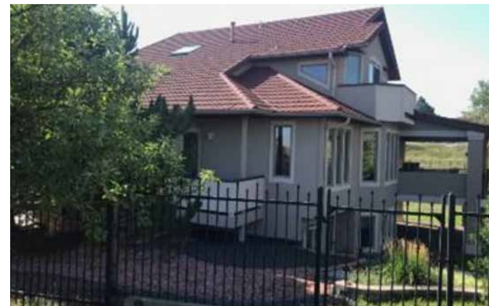
Figure 1.78. Example of metal fence. Where fences are located within 5' of the structure, they should be of noncombustible material such as metal. Image courtesy of Jensen Hughes/FEMA.
