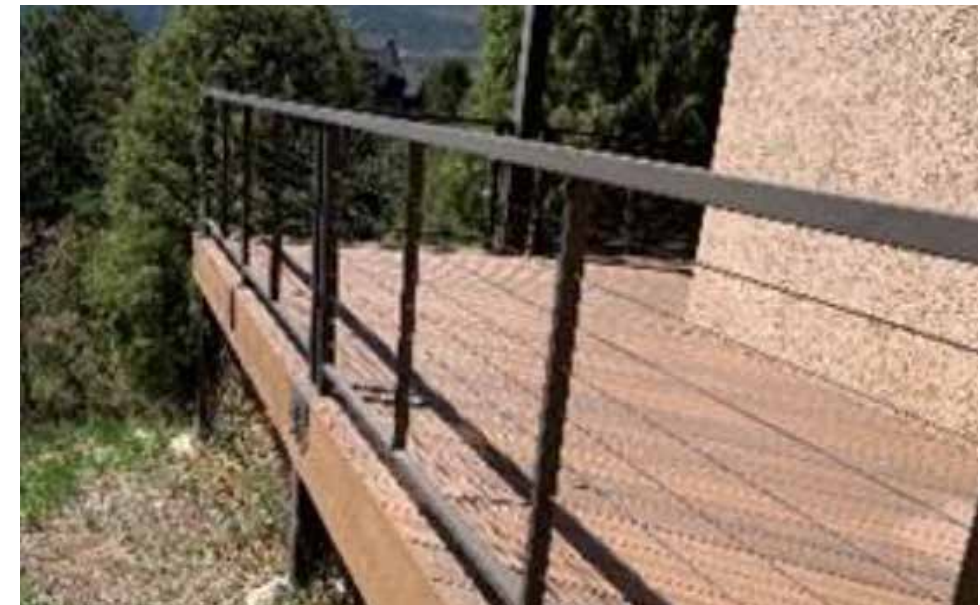
Figure 1.64. Example of deck over sloped ground. Some decks are constructed on sloped ground with unmanaged vegetation near and/or below the deck, exposing the deck and associated home to more severe fire exposure. Image courtesy of Jensen Hughes/FEMA.
