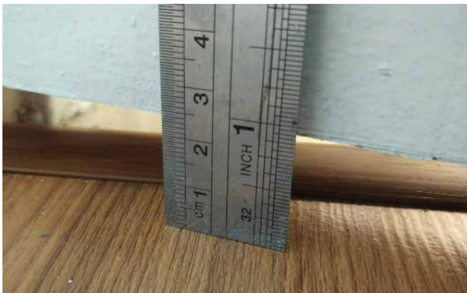
Figure 1.54. Example of gaps in door undercuts. Exterior doors with large gaps at the bottom should be installed with weather strips or replaced.
