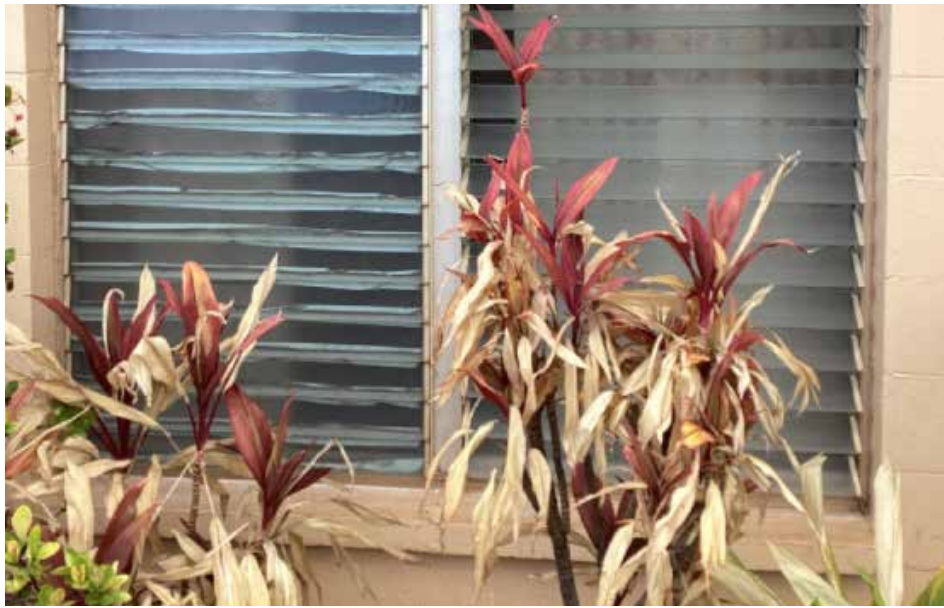
Figure 1.57a. An example of louvered windows with vegetation directly adjacent to the window. Image courtesy of Jensen Hughes/FEMA.
