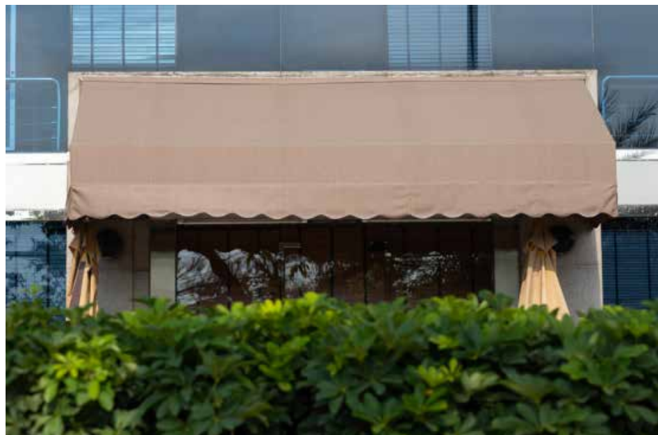
Figure 1.82. Example of canopy. If the canopy material is made of combustible material, the canopy can potentially act as a wick to ignite the home. Additionally, combustible debris can accumulate on canopies configured this way.
