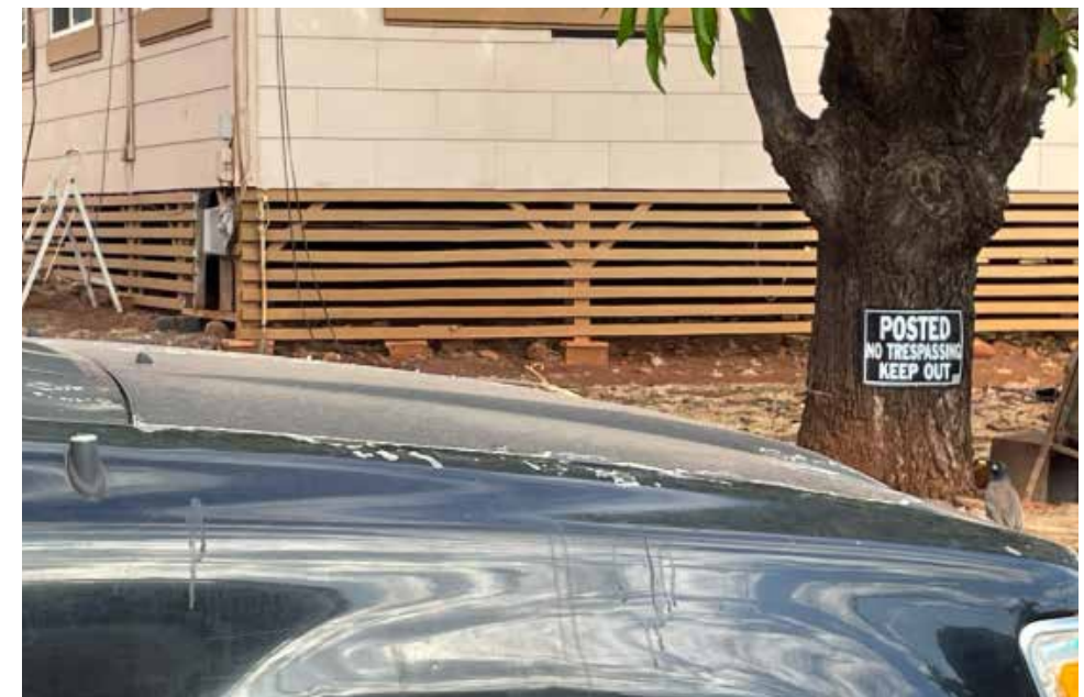
Figure 2.8f. Example of hazardous defensible space with open combustible, post and stilt foundation, which allows vegetative debris and embers to accumulate under the home leading to ignition. Image courtesy of Jensen Hughes/FEMA.
