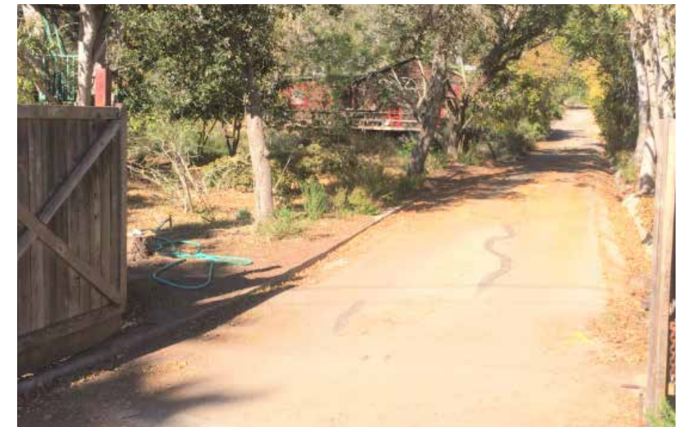
Figure 3.25. Fire access road with insufficient maintenance of hazardous vegetation (roadside and overhead). Image courtesy of Jensen Hughes/FEMA.
