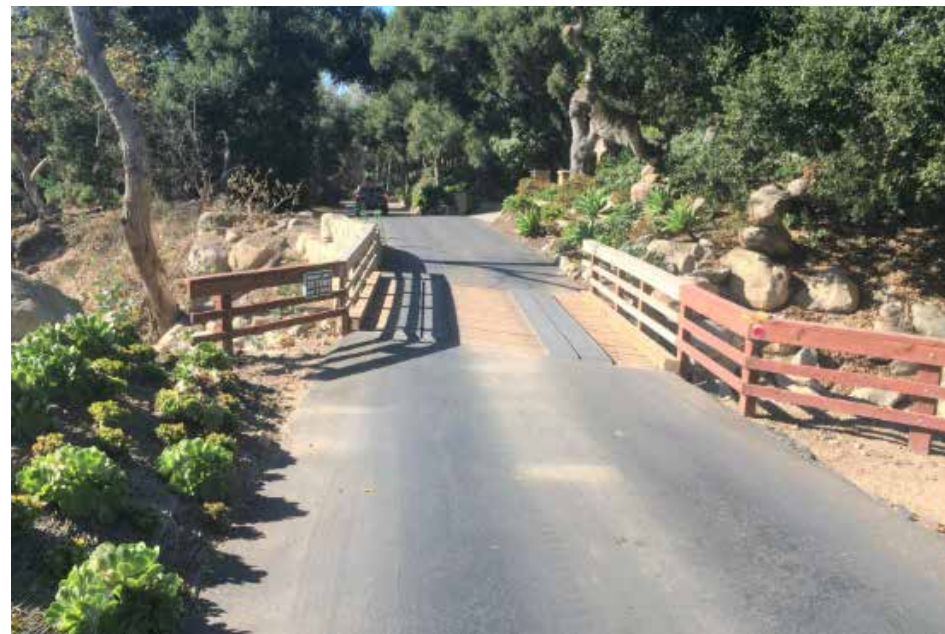
Figure 3.24. Narrow combustible bridge along fire access road. Image courtesy of Jensen Hughes/FEMA.
