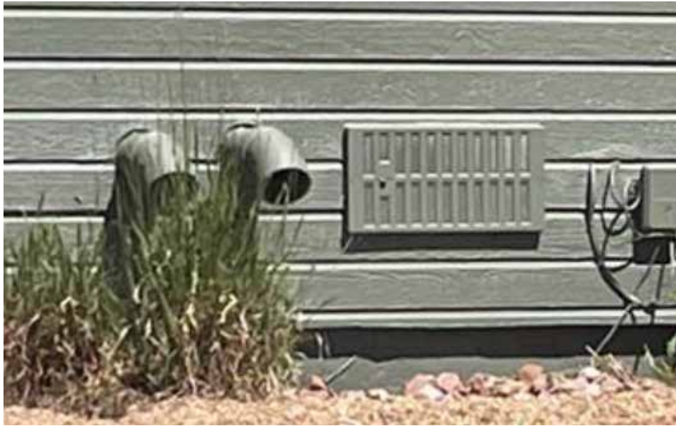
Figure 1.52. Example of vinyl siding. Vinyl siding can melt or burn when exposed to high temperatures and should be avoided. The vulnerability of vinyl siding is increased when flammable materials such as grass and mulch directly abut the home. Image courtesy of Jensen Hughes/FEMA.
