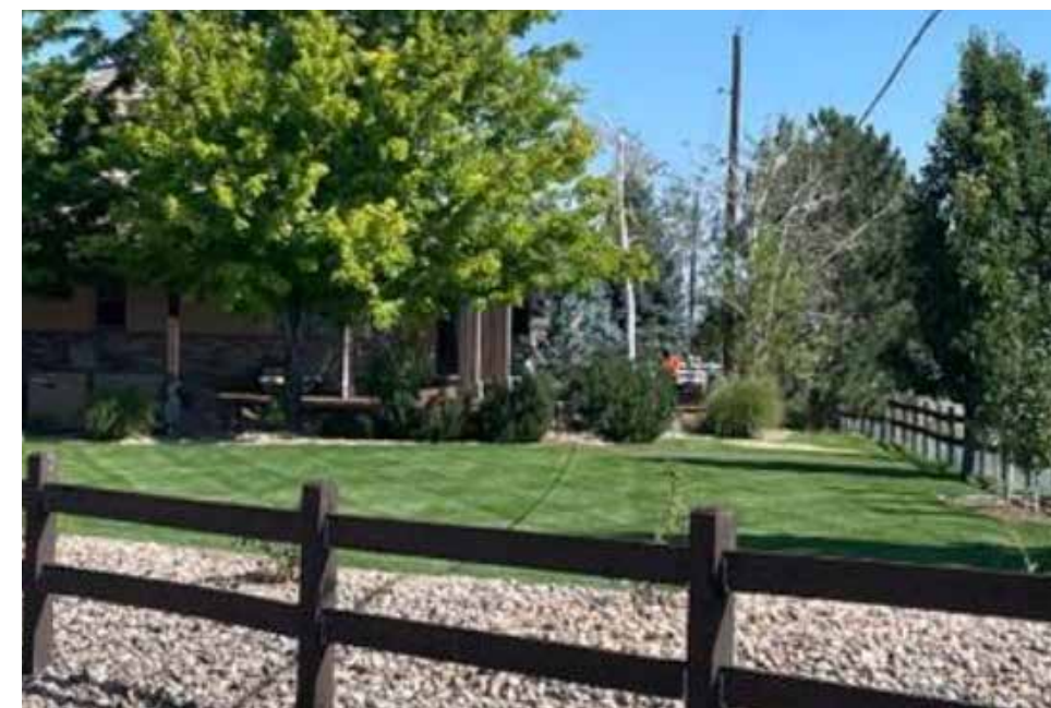
Figure 1.79. Example of cedar split rail fence. Wooden fences present a greater hazard than those of noncombustible materials. Image courtesy of Jensen Hughes/FEMA.
