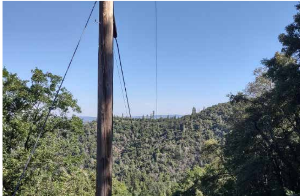
Figure 3.39. Electrical utility infrastructure, particularly aboveground lines and equipment located proximate to hazardous vegetation, challenging terrain, severe weather and remote locations can both cause and be threatened by wildfire. Image courtesy of Jensen Hughes/Tuolumne County.
