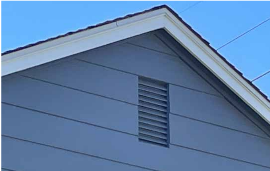
Figure 1.10. Gable-end vent. Gable-end vents such as the one in this photo should be screened. Image courtesy of Jensen Hughes/FEMA.
