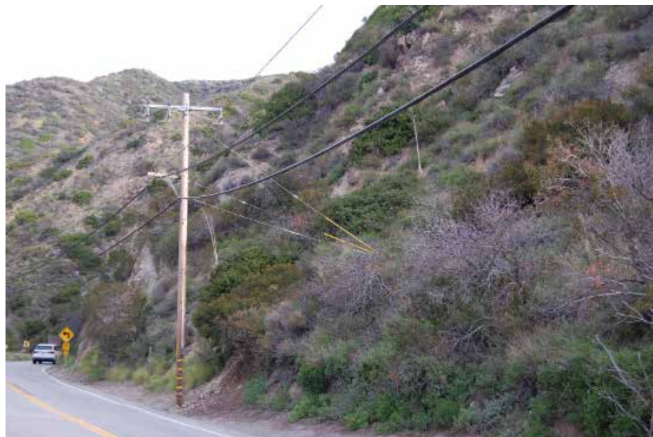
Figure 3.40. Example of a distribution line with unmanaged, dry vegetation in close proximity. Image courtesy of Jensen Hughes/FEMA.
