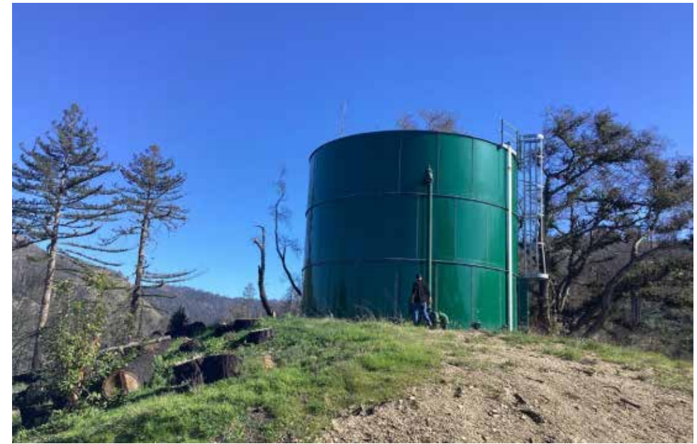
Figure 3.28. Water storage tank located on hill, with vegetation clearance. Image courtesy of Jensen Hughes/FEMA.
