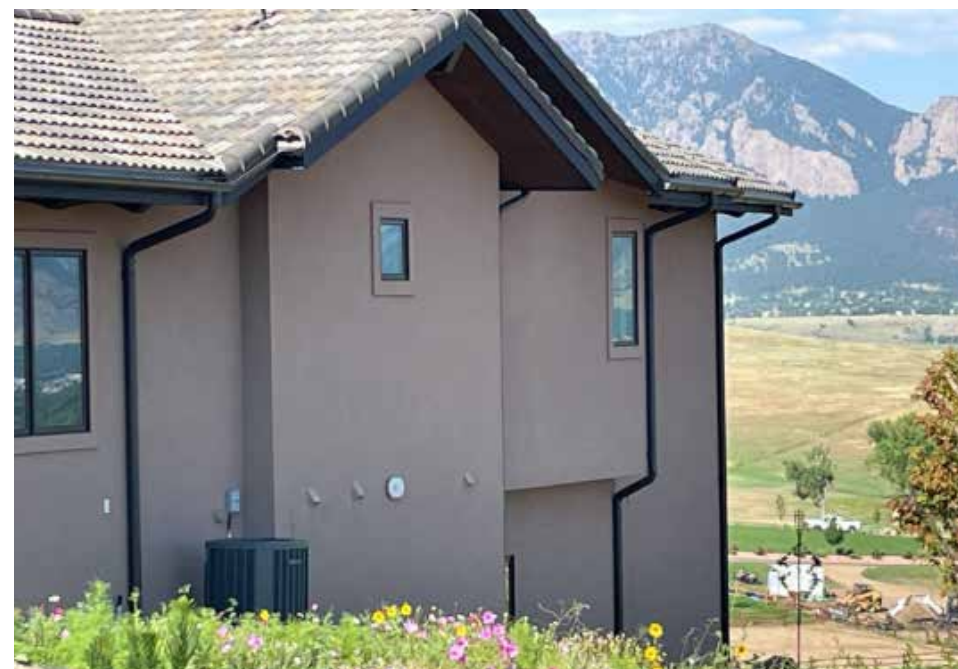
Figure 1.51. Example of stucco cladding. Stucco cladding is one example of noncombustible siding that can be used. Image courtesy of Jensen Hughes/FEMA.
