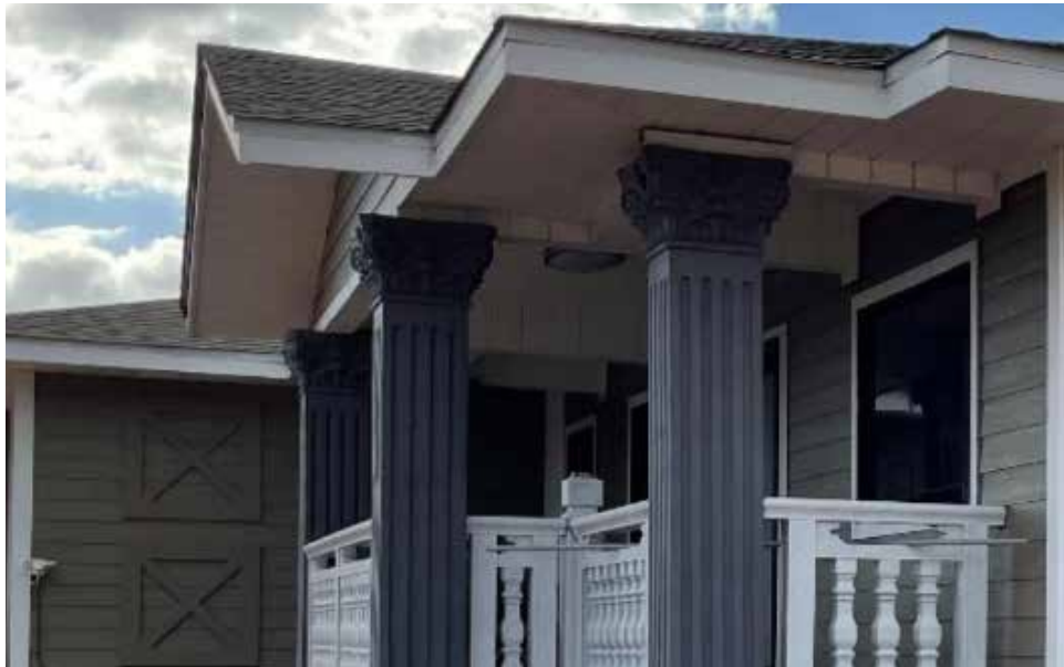
Figure 1.59. Architectural embellishments such as coverings on columns and decorative detailing on exterior wall create additional combustible surfaces where embers and debris collect. Image courtesy of Jensen Hughes/FEMA.
