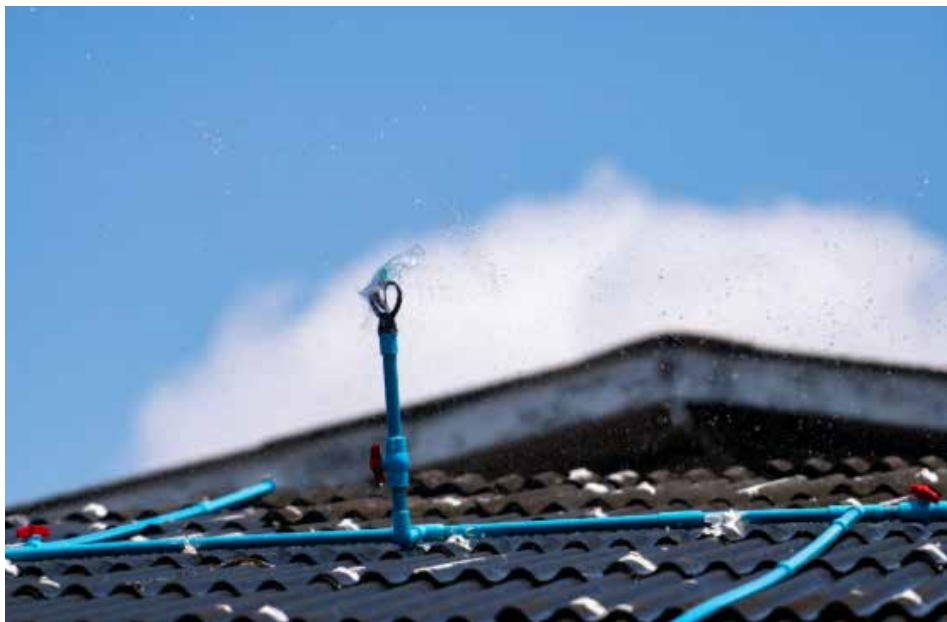
Figure 1.84. Upright sprinkler and piping provided on roof.
