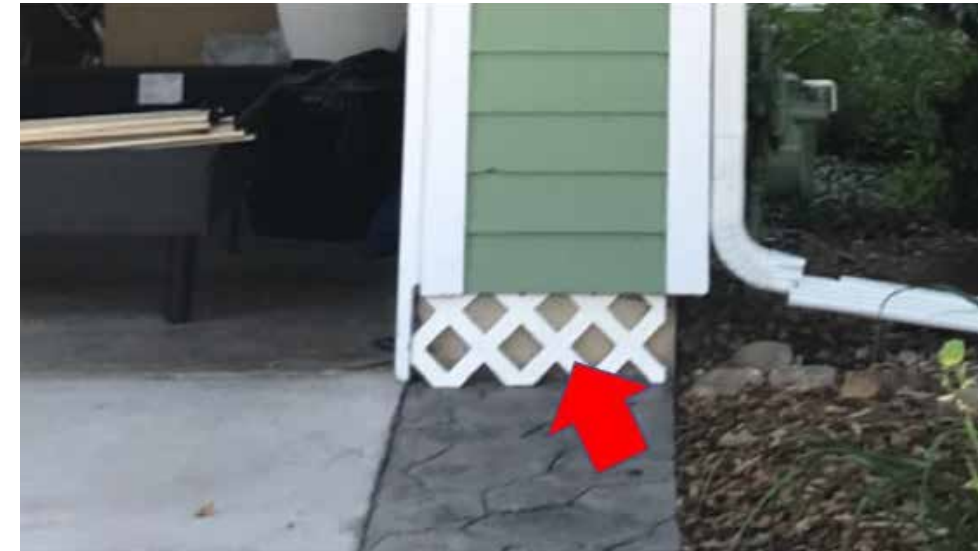
Figure 1.61. This photo shows an example of where adequate bottom-of-wall clearance is provided, but with obstructions. The wooden latticework can provide a path for fire spread. Image adapted from FEMA P-2320, Mitigation Assessment Team Report: Marshall Fire Building Performance, Observations, Recommendations, and Technical Guidance. FEMA, 2023. https://www.fema.gov/
