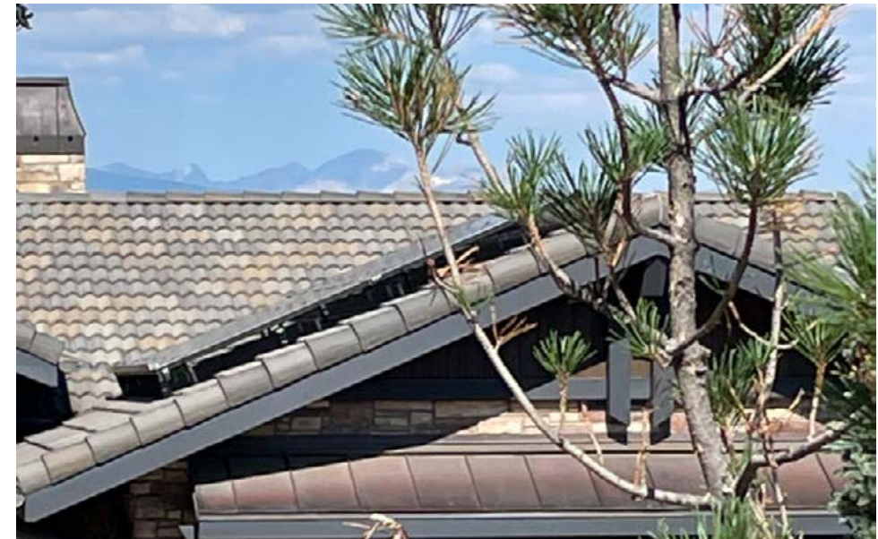
Figure 1.5. Example of composite tile roof. Composite tile roof is one example of a noncombustible roof. However, tile roofs can contain gaps at the ridge line and edges, which should be filled with mortar or bird stop. Image courtesy of Jensen Hughes/FEMA.
