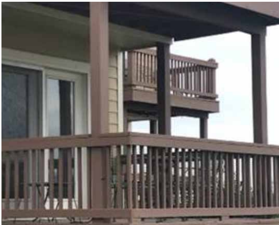
Figure 1.63. Example of single-family residential home with elevated combustible deck. Decks are commonly constructed without an enclosure to limit the placement of combustible goods or vegetation that can provide receptive fuel bed for embers or surface fire. Image courtesy of Jensen Hughes/FEMA.
