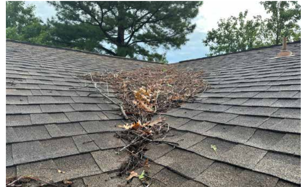
Figure 1.19. Collection of vegetative debris at roof valley joints that create potential fire hazards if ignited by embers. A localized fire can readily penetrate an unprotected joint.
