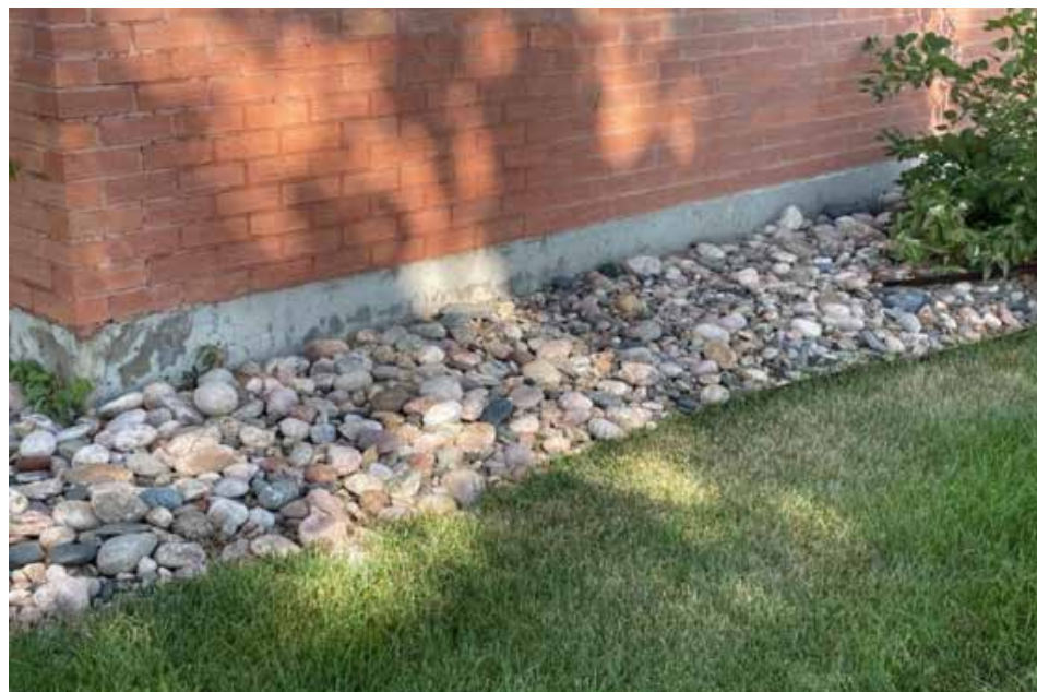
Figure 2.10. Example of enhanced, non-combustible Zone 0 (0-5') 6" of non-combustible bottom-of-wall detail, well maintained grass and shrubs. Image courtesy of Jensen Hughes/FEMA.
