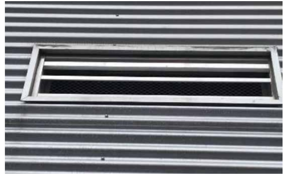
Figure 1.53. Example of corrugated steel siding on exterior wall. Corrugated steel siding is a good noncombustible exterior cladding option, however care should be taken to ensure there are no gaps between steel siding panels. Image courtesy of Jensen Hughes/FEMA.
