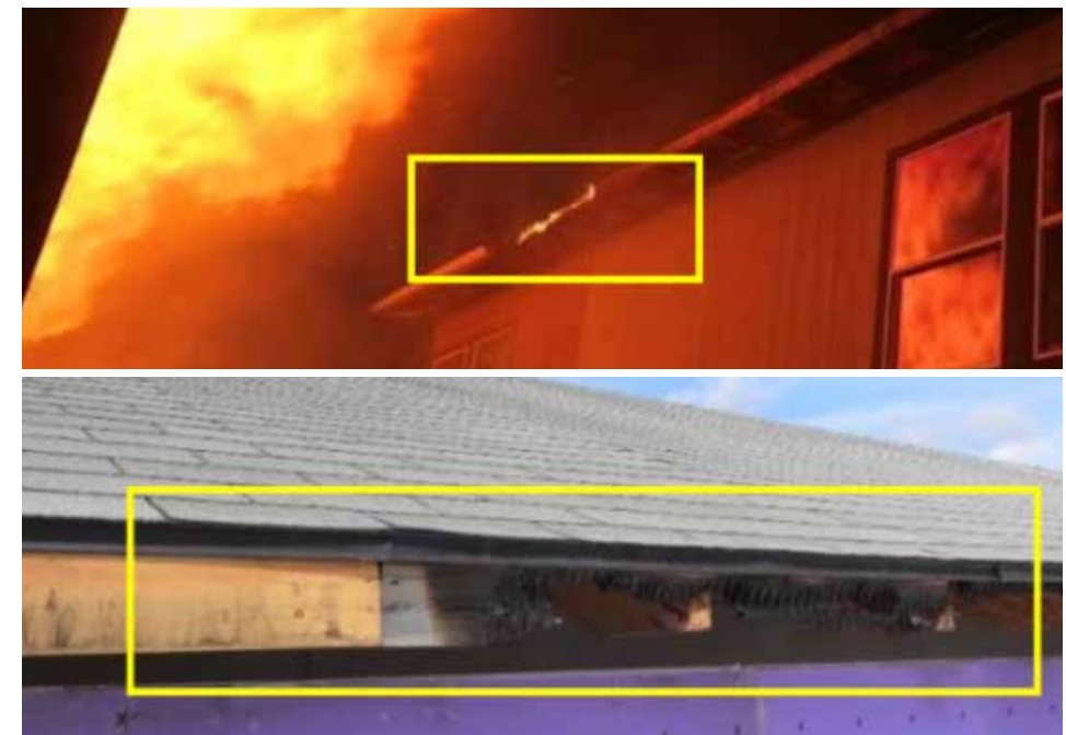
Figure 1.28b. Example of fascia and roof edge that ignited, and began burning roof construction. Image courtesy of Jensen Hughes/FEMA.
