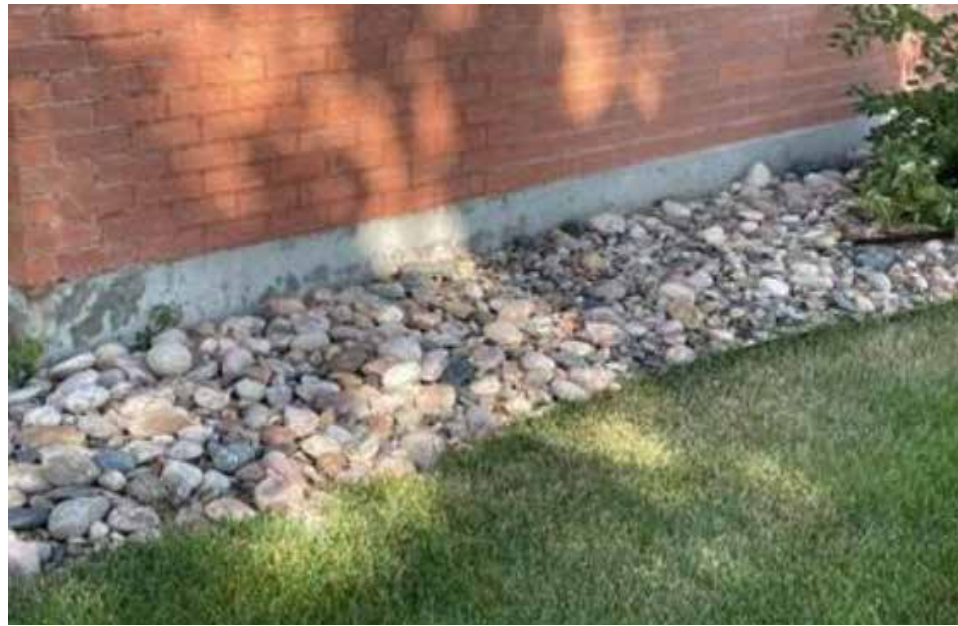
Figure 2.9. Example of ember-resistant Zone 0 (0-5') with 6" of non-combustible bottom-of-wall detail, hardscaping, minimal vegetation and well-maintained grass and shrubs. Image courtesy of Jensen Hughes/FEMA.
