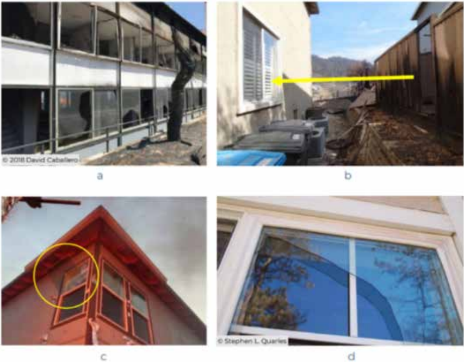
Figure 1.57b. Four examples of window vulnerabilities. Image adapted from Wildland Fire Embers and Flames: Home Mitigations That Matter, IBHS, 2023. https://ibhs.org/risk-research/wildfire/
