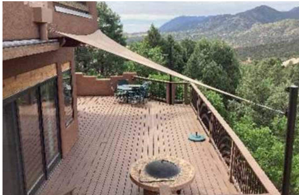
Figure 1.81. Example of patio covering that provides a potential source for debris and ember collection. The covering should be of ignition-resistant materials. Image courtesy of Jensen Hughes/FEMA.
