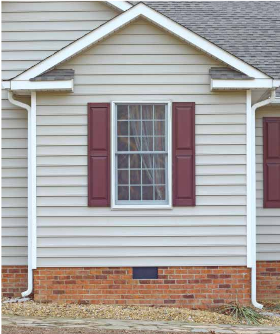
Figure 1.75. Example of brick foundation below siding. While brick is a non-combustible material and there is less of a concern of a surface fire breaching the home via the foundation, it is important to note that the foundation shown still contains vents that must be protected.
