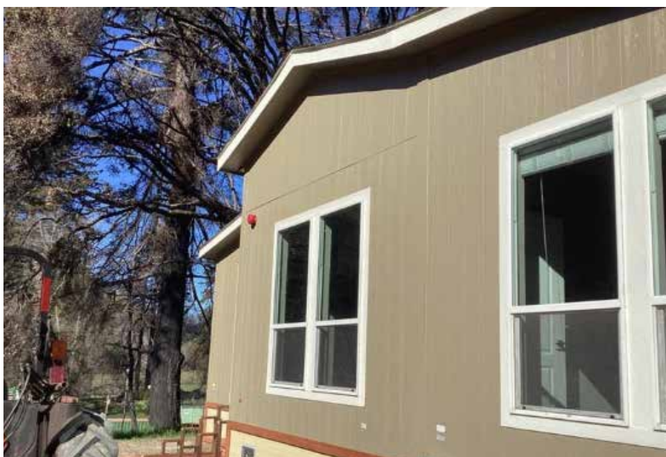
Figure 1.50a. Example of fiber cement board cladding on exterior wall. Image courtesy of Jensen Hughes/FEMA.
