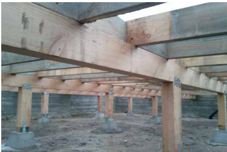
Figure 1.72. Example of an open pier and stilts foundation. This photo shows combustible covering around the open foundation, which presents a hazard to the home. Image by RBerteig on Flickr., CC BY 2.0.
