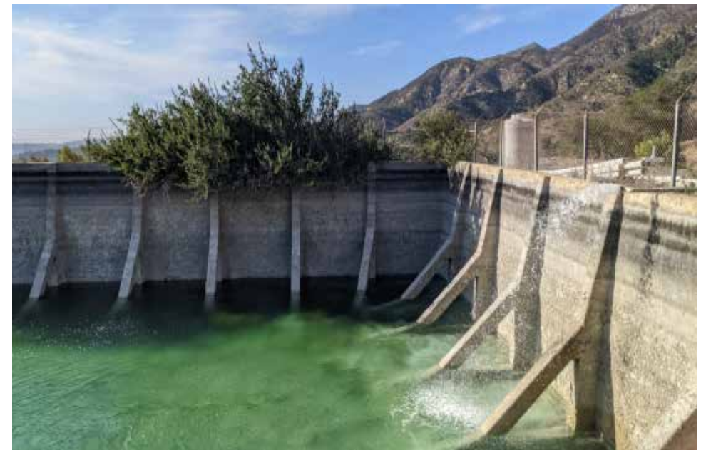
Figure 3.33. Large water reservoir, filling automatically, serves private gravity fed system. Image courtesy of Jensen Hughes/FEMA.
