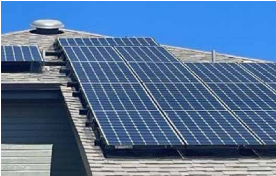
Figure 1.17. Solar panel array on roof. Configurations such as the one shown are prone to debris accumulation under the array. Image courtesy of Jensen Hughes/FEMA.
