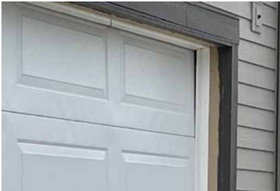
Figure 1.55. Example of gaps around garage door. These gaps can lead to potential ember intrusion or ignition of the frame of the garage door, if combustible. Image courtesy of Jensen Hughes/FEMA.
