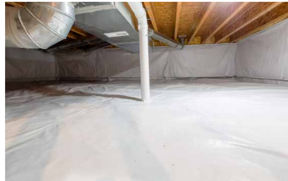
Figure 1.73. Example of a crawl space foundation. Crawl space foundations typically contain vents that are susceptible to ember intrusion.
