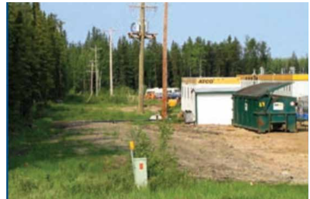
Figure 3.42. Example of tree removal clearance around distribution lines. Image reused under the Open Government - Alberta License https://open.alberta.ca/licence
