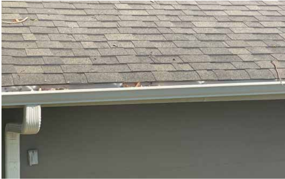
Figure 1.33. Debris in gutters (as pictured) can ignite and lead to ignition of the sheathing and fascia board. Image courtesy of Jensen Hughes/FEMA.
