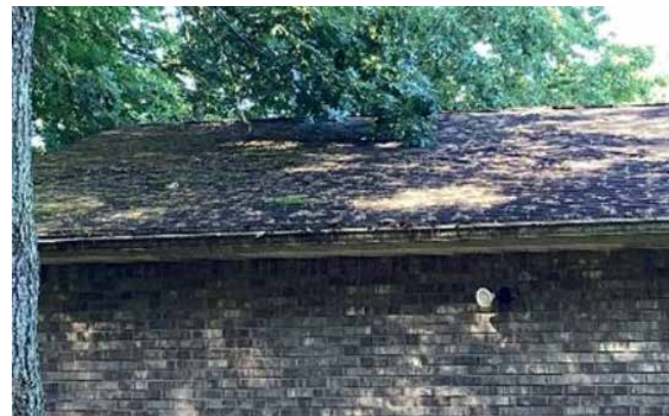
Figure 1.36. Heavy debris loading in gutter and on roof. This is caused by the overhanging vegetation. Where possible, overhanging vegetation should be removed to lower the severity of debris accumulation. Image courtesy of Jensen Hughes/FEMA.
