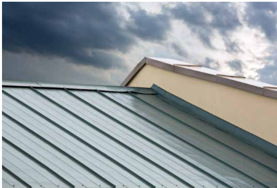
Figure 1.47. Example of metal flashing at a bottom-of-wall-to-roof joint.
