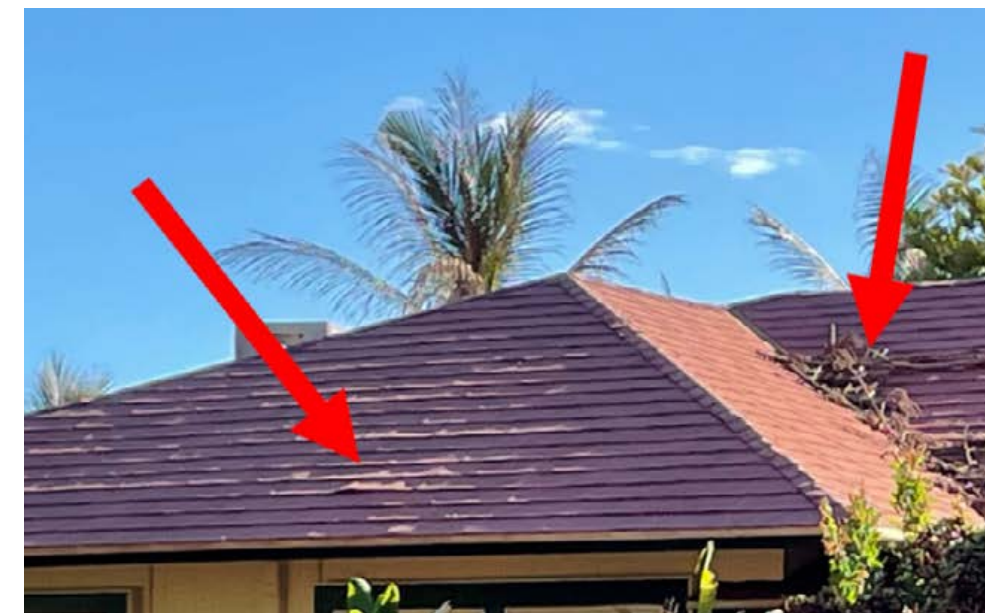
Figure 1.2. Examples of roof construction vulnerabilities (Red arrows indicate debris accumulation (right) and curled shingles (left)). Image courtesy of Jensen Hughes/FEMA.
