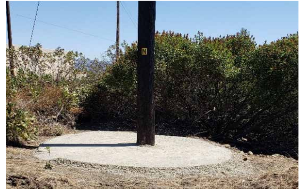
Figure 3.41. Example of 10' vegetation clearance around a distribution pole. Image courtesy of Jensen Hughes/FEMA.
