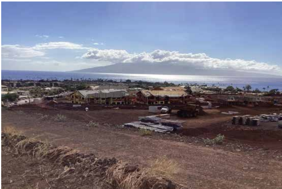
Figure 3.22. Example of a residential development under construction, where light frame timber construction and staging areas with combustible materials pose potential sources of ignition during a wildfire. Image courtesy of Jensen Hughes/FEMA.
