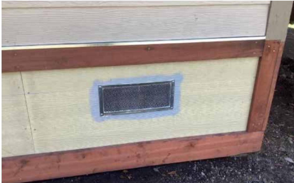
Figure 1.66. Example of crawl space vent. Crawl space vents are a vulnerability in wildfires if unprotected, as they are oftentimes located proximate to dry grasses, vegetative debris, mulch or other ornamental landscaping. Image courtesy of Jensen Hughes/FEMA.
