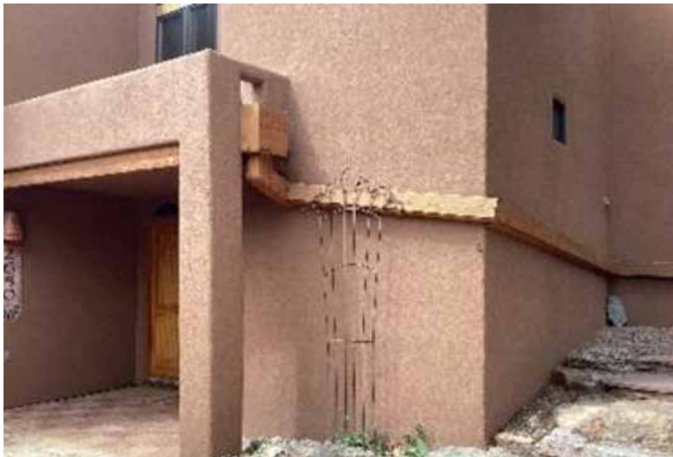
Figure 1.60. Decorative balconies and overhangs. These types of architectural embellishments are prone to combustible debris accumulation. Image courtesy of Jensen Hughes/FEMA.
