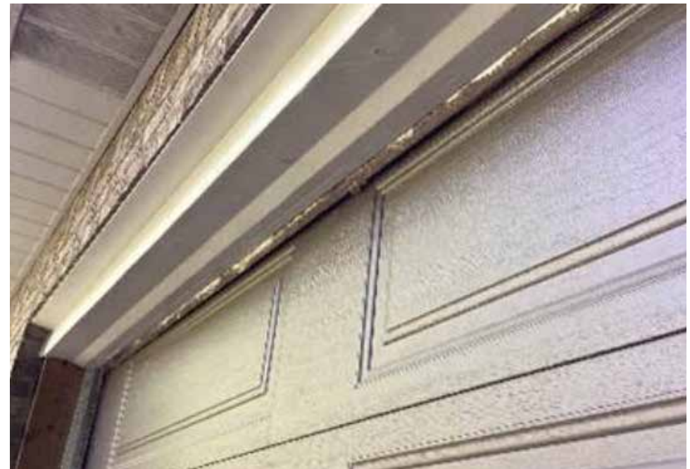
Figure 1.56. Example of gaps around garage door. These gaps can lead to potential ember intrusion or ignition of the frame of the garage door, if combustible.
