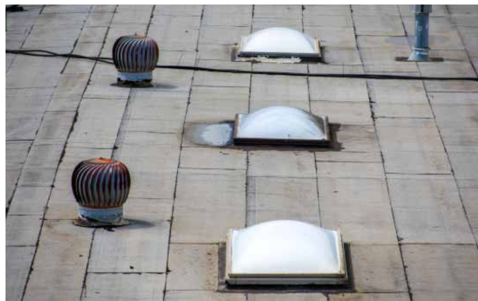
Figure 1.13a. Example of flat roof with plastic dome-type skylights. Flat roof skylights are vulnerable to combustible debris accumulation, as well as gaps in the joints between the skylight and the roof. Note also the turbine vents to the left of the skylights.
