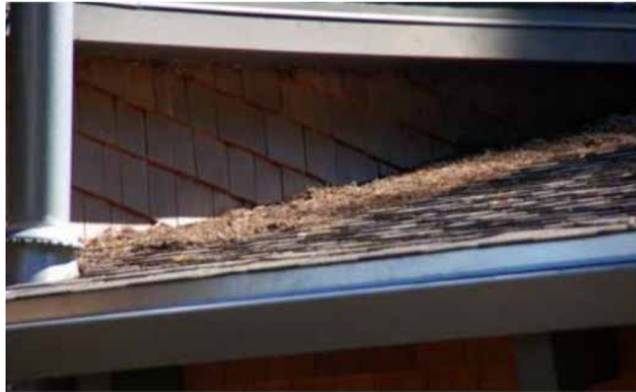
Figure 1.20. Collection of vegetative debris at roof-to-wall joints that create potential fire hazards if ignited by embers. Accumulated debris can be ignited by embers and ignite the combustible siding where the exterior wall meets the roof. Image courtesy of Stephen Quarles.
