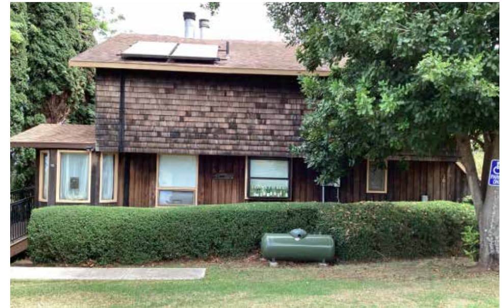
Figure 2.8e. Example of hazardous defensible space with dense shrub, hazardous trees (e.g., Italian cypress), overhanging trees, and propane tank within Zone 0 (0-5 feet) and Zone 1 (5-30 feet), in combination with wood shake single siding. Image courtesy of Jensen Hughes/FEMA.
