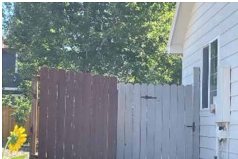
Figure 1.77. Example of cedar privacy fence attached to house. Any fencing that directly connects to the home should be replaced with noncombustible material for at a minimum 5' within the vicinity of the home. Image courtesy of Jensen Hughes/FEMA.
