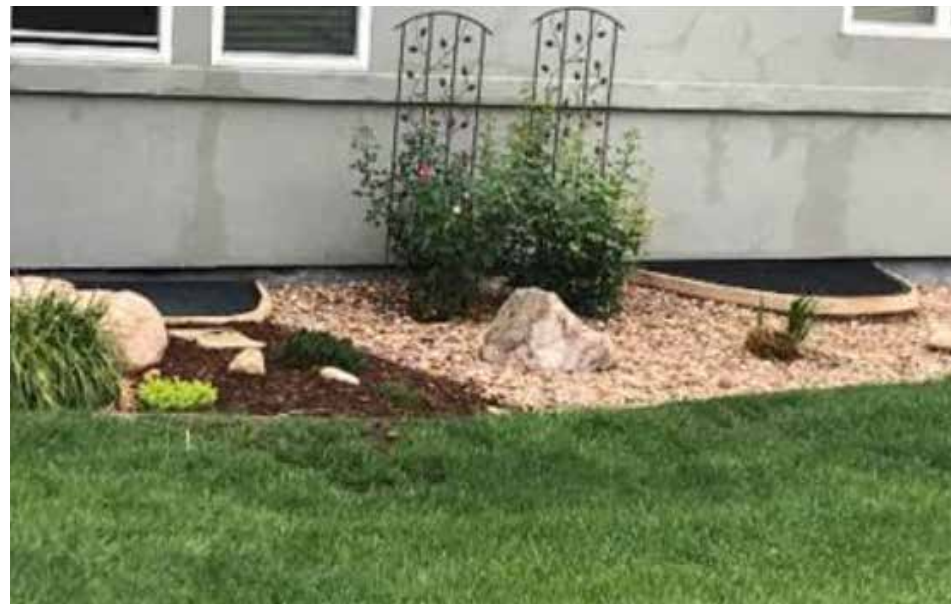
Figure 1.68. Example of light well that is hardened. Noncombustible grates are one way to prevent combustible debris from collecting in the window well. Image courtesy of Jensen Hughes/FEMA.
